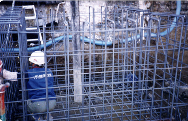
High rebar density increases construction difficulty
