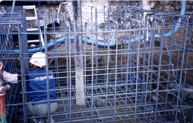
High rebar density increases construction difficulty
